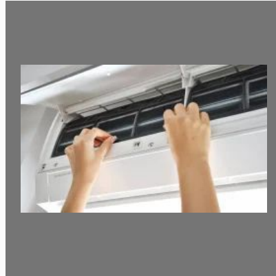
Blue Star Air Conditioner Repairing Service
