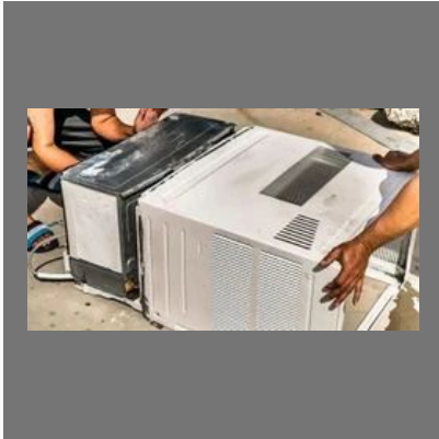
Window Air Conditioner Repairing Service
