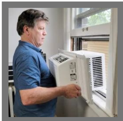
Window Air Conditioner Installation Service
