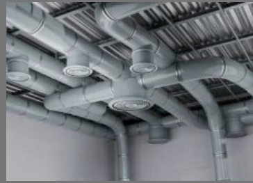
HVAC PVC Pipe Installation Services
