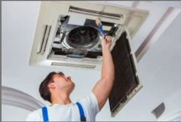
HVAC Equipment Installation Services
